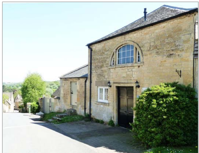
Blockley Little Village Hall - external view
